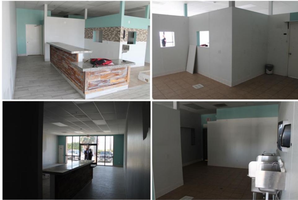
Current condition of the unit
